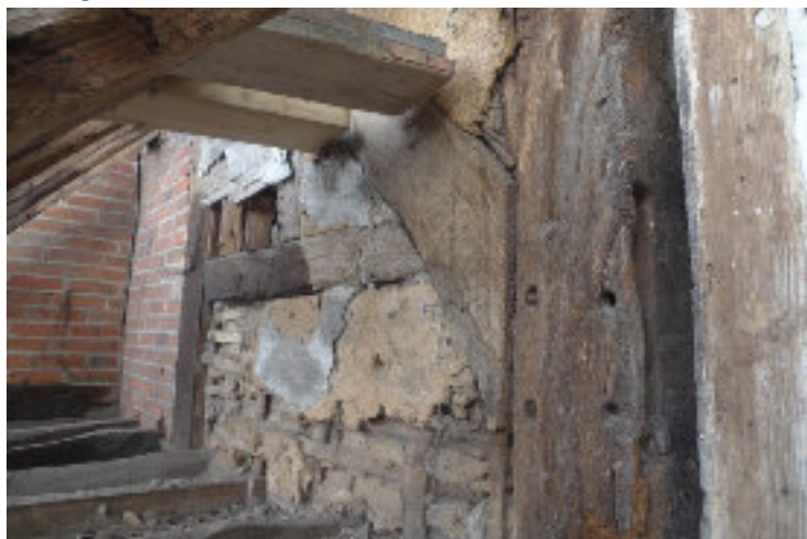
FIG. 3 Rear of bay DE showing mullion window during renovation.
