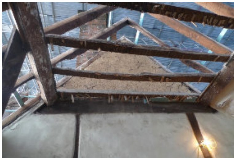
FIG. 7 Above left: Apex of roof on east side of truss D. This shows that above collar level it was never plastered, as it was not meant to be seen. The chamber next to the smoke bay must therefore have been ceiled at collar level from the outset.
