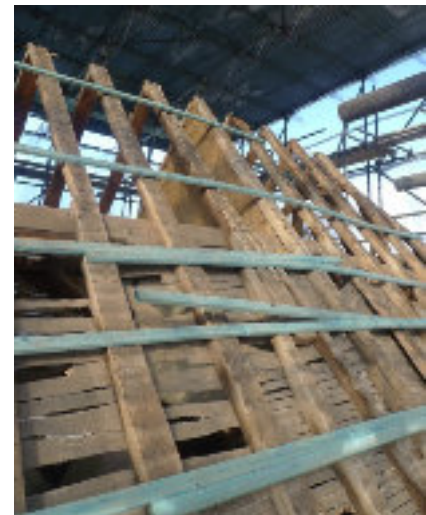
FIG. 7 Above left: Apex of roof on east side of truss D. This shows that above collar level it was never plastered, as it was not meant to be seen. The chamber next to the smoke bay must therefore have been ceiled at collar level from the outset.
