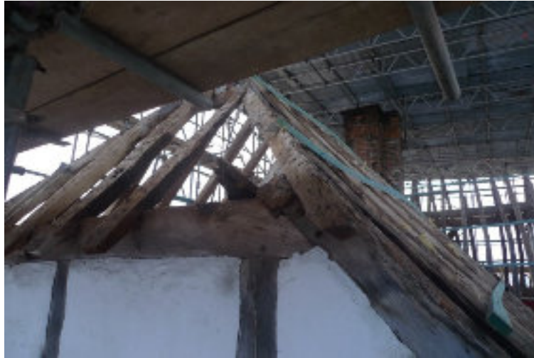
FIG. 5 Framing for the half hipped roof at the east end of the original house.
