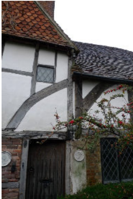
FIG. 2 Left: Separate framing of original house and later cross wing.
