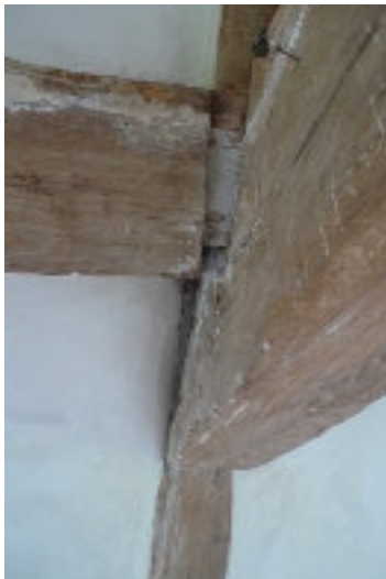
FIG. 13 Left: The purlin of the cross wing roof, halved to fit into the collar.
