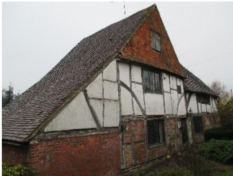
Photo of Yew Tree Cottage in 2015 before conservation and extension works
