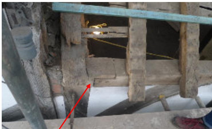
FIG. 4 Above: Scarf joint at post D
